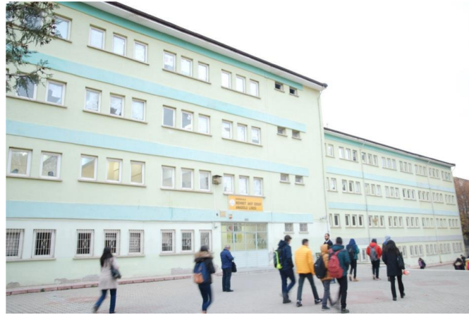
Figure 10. Front view of the building
